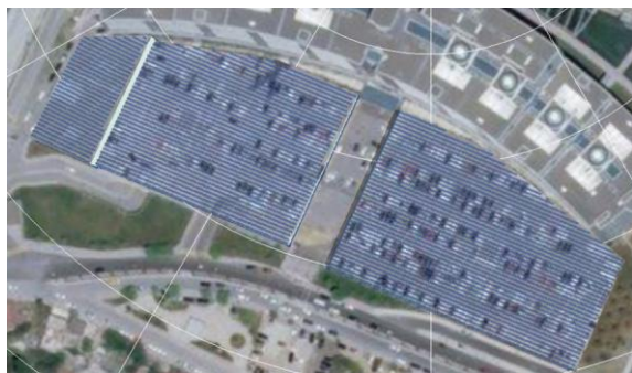
Fig. 10. Mounting the modules on car parking area.
