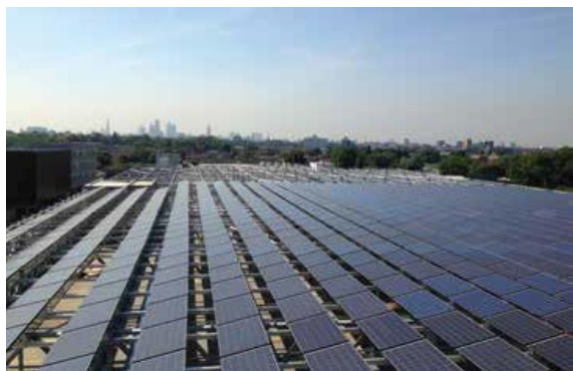
Fig. 11. The canopy type photovoltaic system for car parking area.
