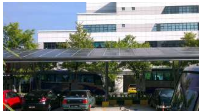
Fig. 8. The 17.28 kWp solar PV carport system.
