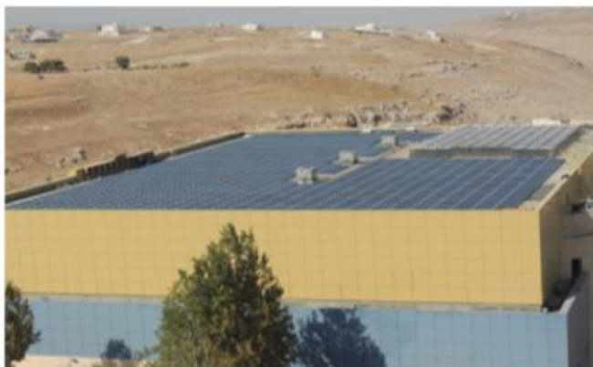
Figure 2. PV plant on the roof of Cultural Foundation Forums Building (ARENA) in AAU, Amman, Jordan
