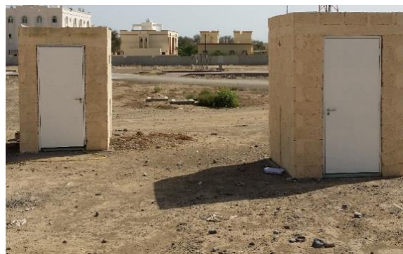
Fig. 1. Identical test rooms.
