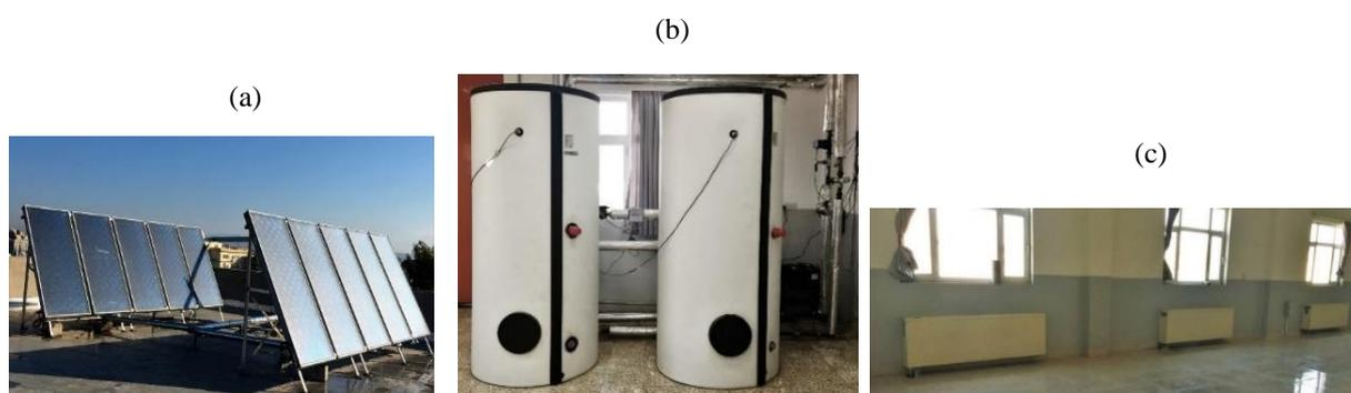
Fig. 3. Main components of SWHS: (a) solar collectors, (b) storage tanks, and (c) fan coil units.
