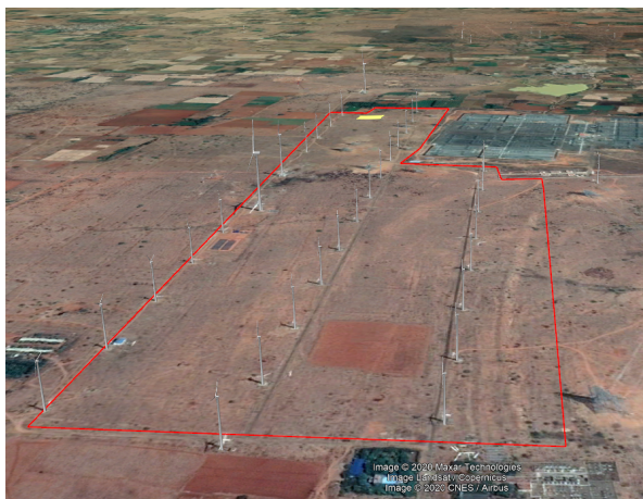
Fig. 6. Layout of one-on-one wind turbine substitution for 200 kW with 250 kW capacity at exactly the same coordinates (Google map)
