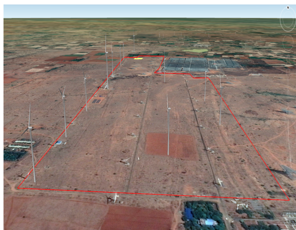
Fig. 7. Layout of substitution of old 200 kW wind turbines with a capacity of 850 kW wind turbine (Google map)
