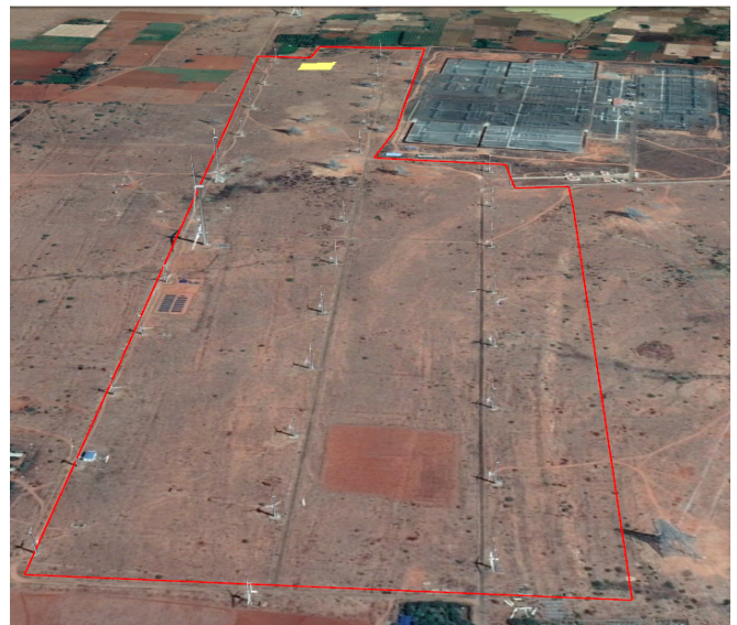
Fig. 5.a. The repowering layout of existing operational Kayathar wind farm (Google map)
