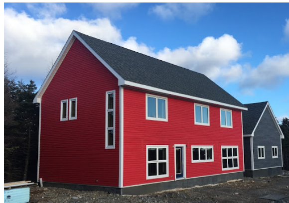
Fig. 1. First house built on PHIUS+2015 standards in Newfoundland.
